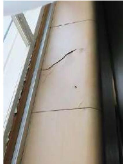
An example of damage to the leather panels due to exposure to light and heat, as a result of their proximity to a window
