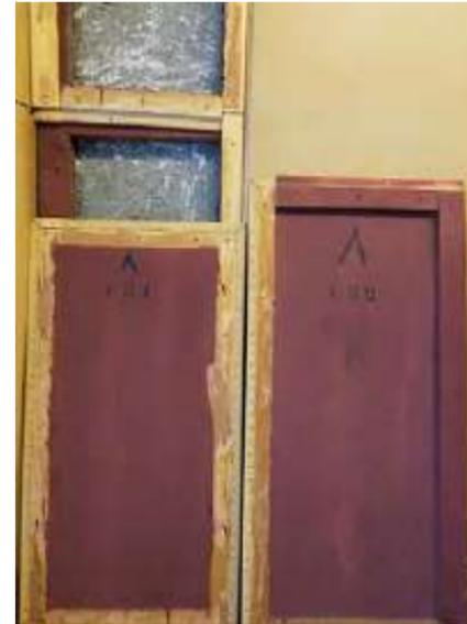
Before the renovation works began, three panels were removed to study their construction and mounting; each panel is numbered on the back.
